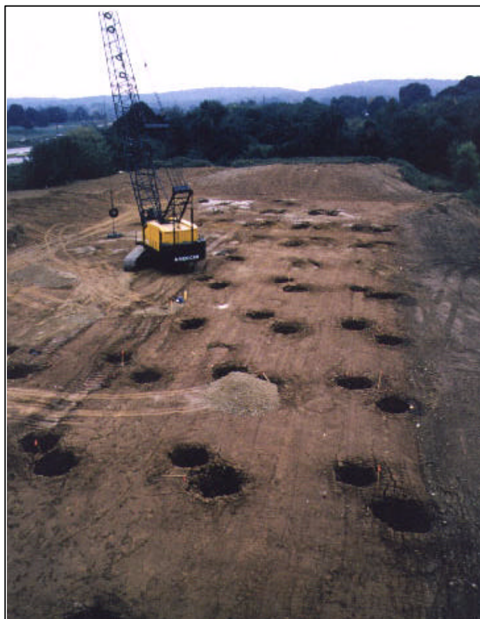
Fig. 3 – Valley Forge building site
